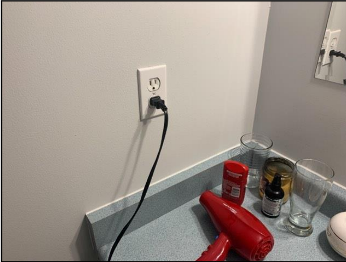
12. GFCI - basement bathroom
