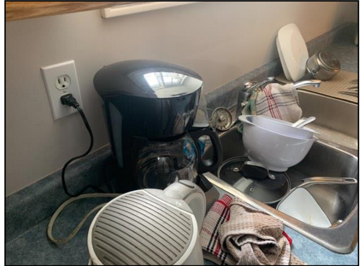
13. GFCI - basement kitchen
